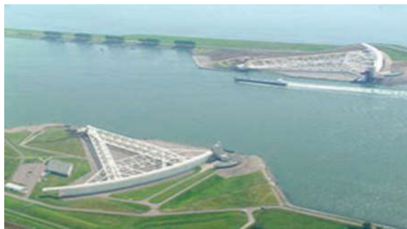
Fig. 12. Netherlands North Sea Protection Works
